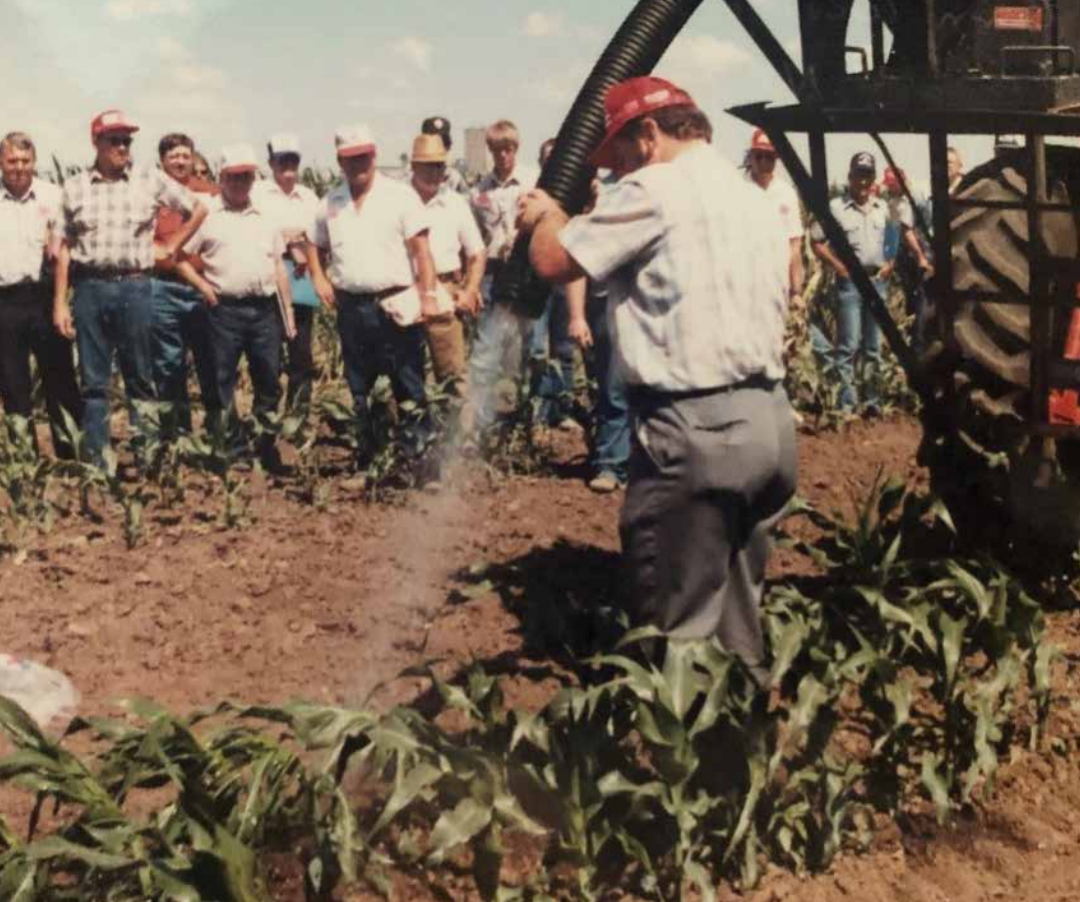
Imitating hail with an ice blowing machine. The crop insurance industry funded the development of these machines in the 1980's to create realistic crop damage for loss adjuster schools and they are still in use today.
